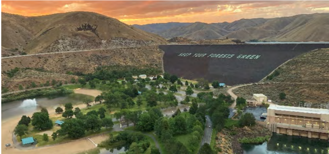
LUCKY PEAK DAM, IDAHO (WALLA WALLA DISTRICT)
